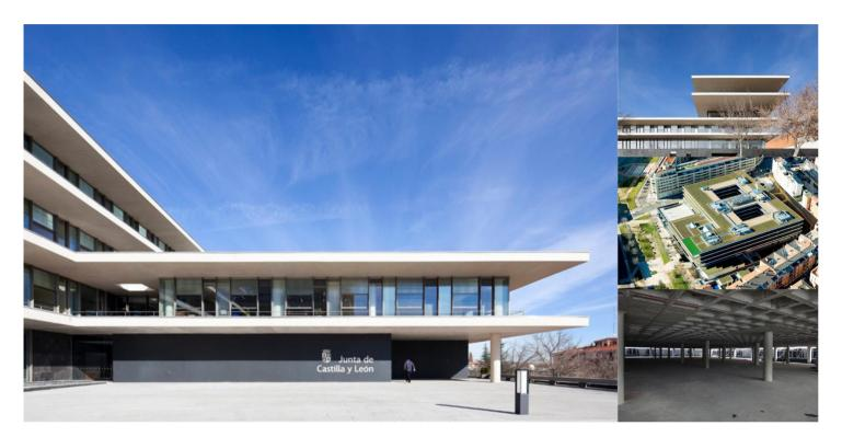
The building offers a singular architectural and engineering design both for its large 14.0m spans, creating large diaphanous areas which have enormous functional potential, as well as for its external white concrete finish on the wings, whose spans stretch out from between 2 to 7 meters.
